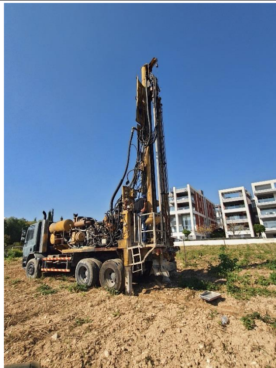
SCHRAMM Drilling Rig used for intrusive investigations
