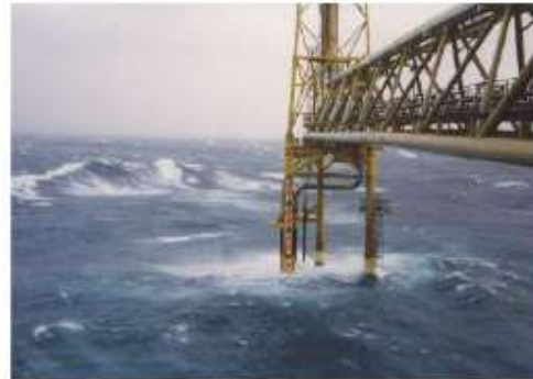
A major application area of MIKE 21 SW is in connection with design and maintenance of offshore structures
