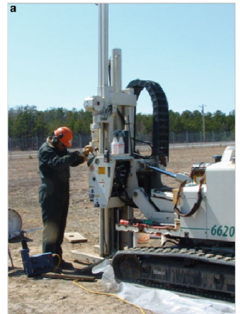
Picture 1 : In situ chemical Oxidation (ISCO). Injection Method : Direct push injection (during drilling)
