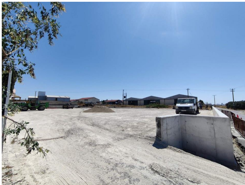
Figure 40: Construction near the area
